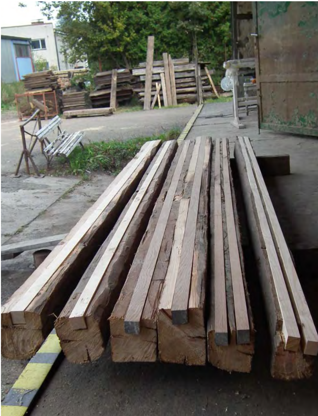
Fig. 1: Timber members damaged by ligniperdous insect with embed reinforcing core
